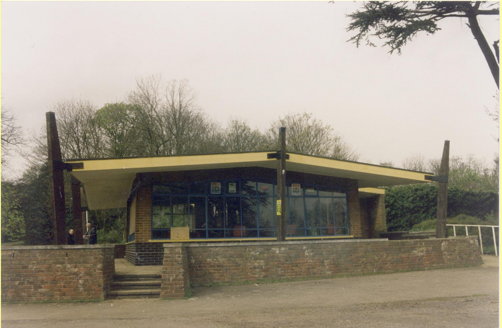
The old visitor centre at Bedfords photographed in 1998. It was a tired and redundant building barely thirty years after it opened in 1964
